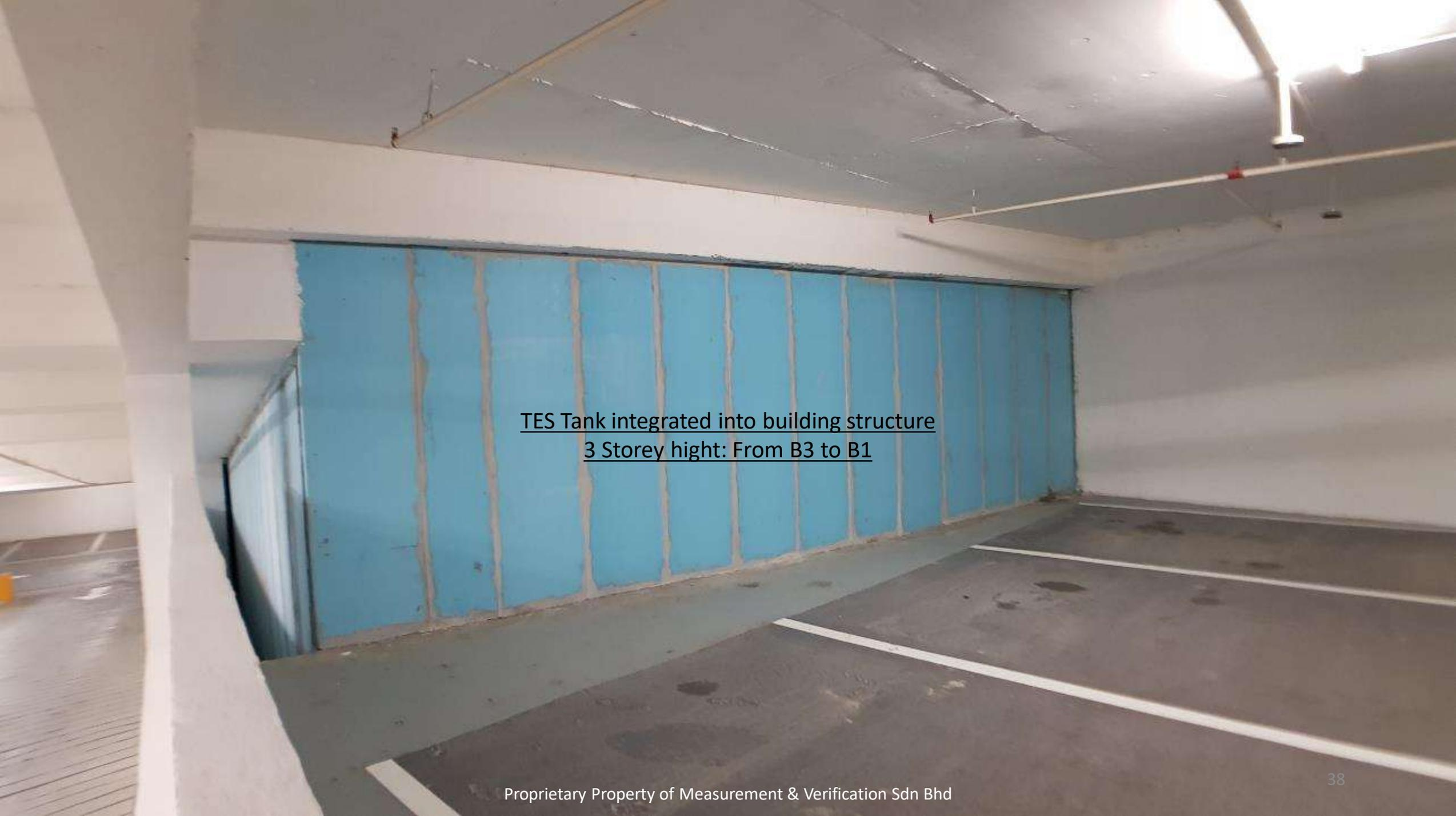
TES Tank integrated into building structure
